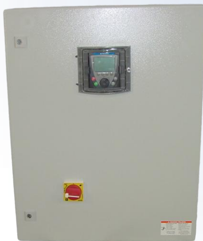
10 HP ELECTRICAL ENCLOSURE FOR VFD/BLOWER
